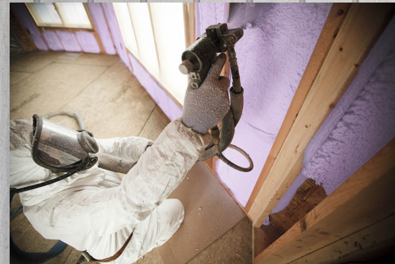
Closed Cell Spray Foam Wall Insulation Option
